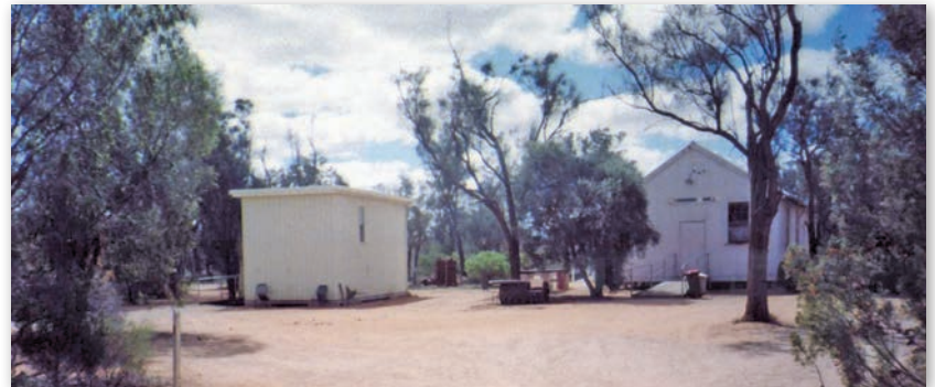
Inside the park showing hall and telecom building
